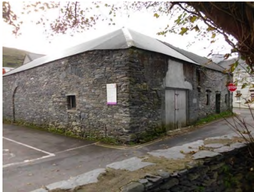
Cahirciveen Penal Church and Schoolhouse, a National Monument. Now decommissioned and used as a mechanic's workshop.
